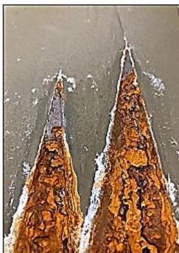
Close up of right of Q42 after 72 hrs of exposure
